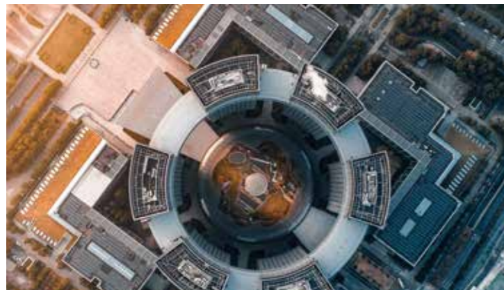
1.2MW ☰ Hangzhou Civic Center Podium Roof Photovoltaic Power Station 📍 Hangzhou, Zhejiang Province, China
